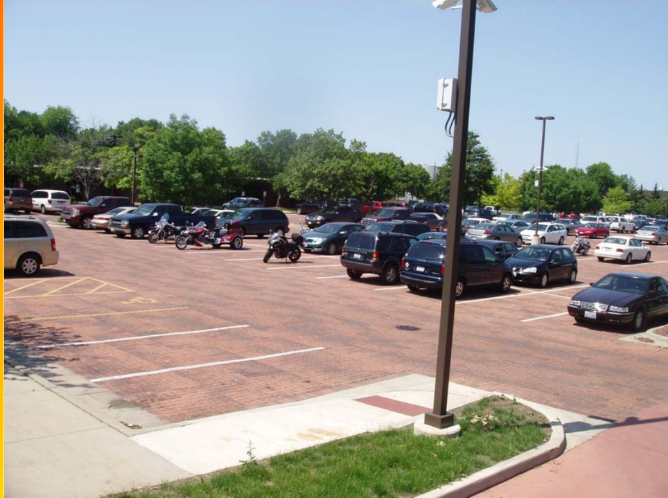
Pervious concrete paver parking lot at Champaign-Urbana MTD building.
