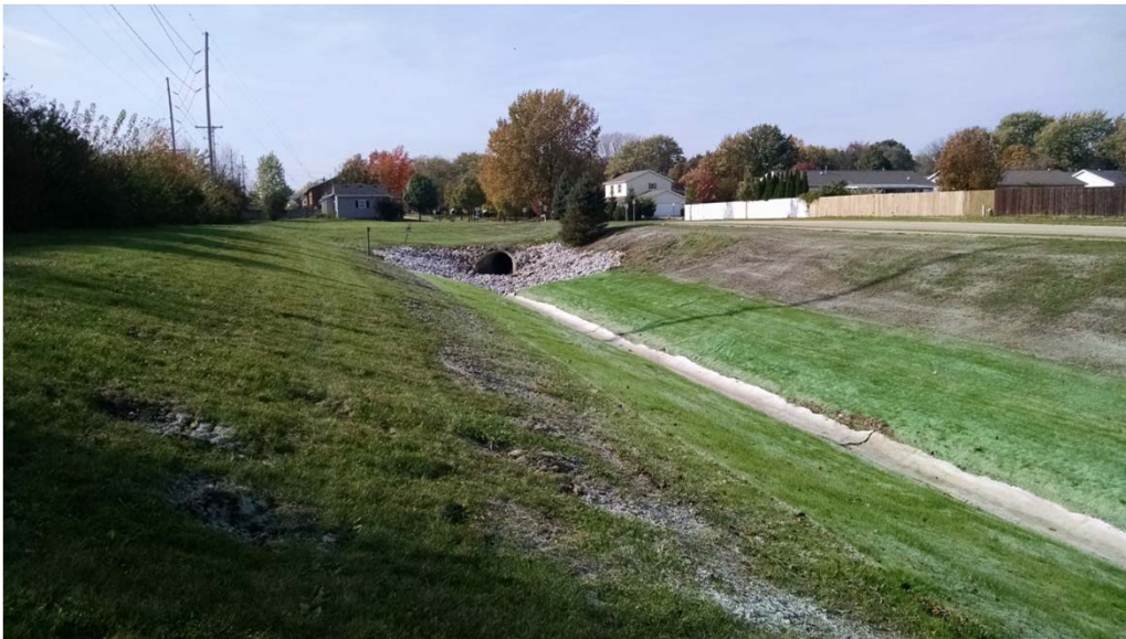
Fairway Estates Detention Basin Improvements
