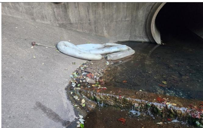
Sediment sock has broken loose from its second anchorage point and was moved to the side.
